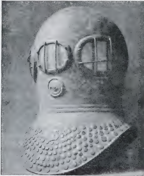
FIG. 12.—SIEBE'S FIRST DIVING HELMET.
